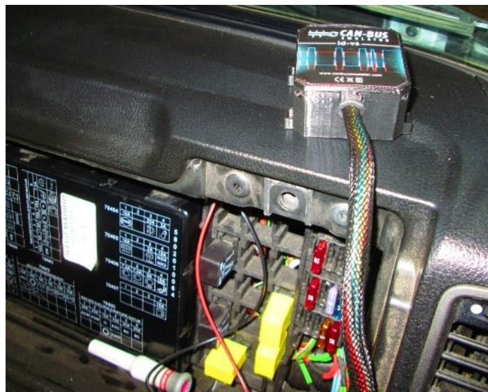
Figure 24 Visual inspection: Fuse Box
