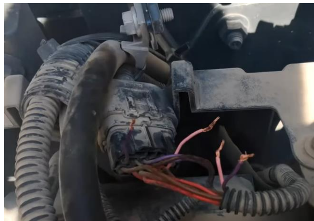
Figure 4 USM isolated after urea pump and pressure signal wiring cut
